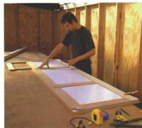
Template defines the countertop's shape. A template (top photo) made of thin plywood strips hot-glued together is an accurate means of transferring the shape of the counter onto the mold. After notations are written on the template indicating site particulars, the template is flipped over (remember, the mold is upside down), and the information is transferred onto the melamine blank (bottom photo).
